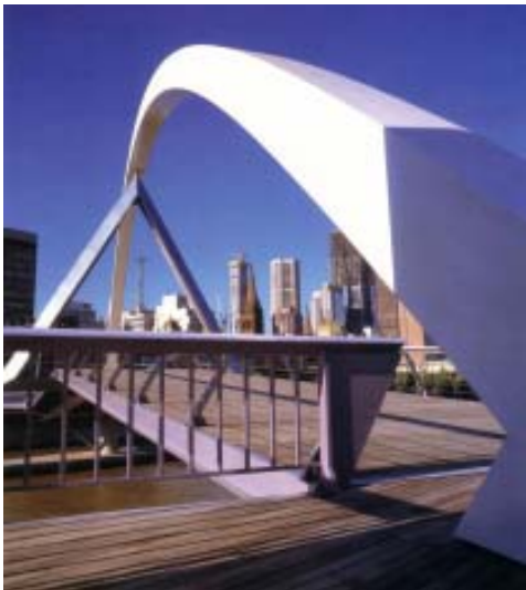
Yarra River Pedestrian Bridge
